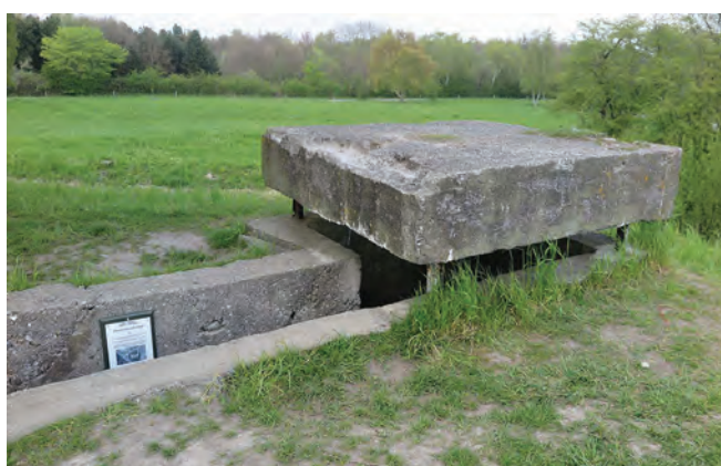
Observation bunker at Kongelunds Fort
